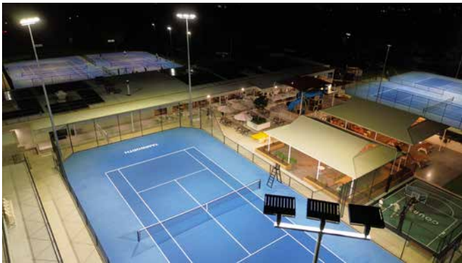
480W, 720W and 960W STRIKER Sports Lights on new and existing poles, producing over 350 lux over 4 standard courts with 8m poles, 500 lux over 6 courts with 12m poles and 1000 lux over the ITF competition court for TV broadcasting. Note the uniformity of illumination of the courts and surrounds, with minimal light spill into adjacent non-pedestrian areas.
