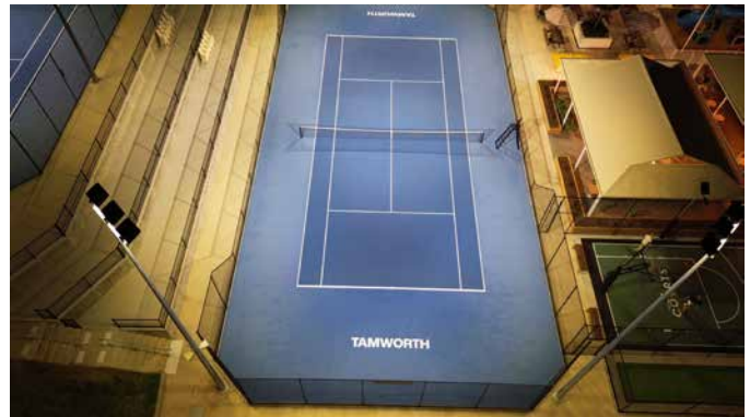
480W, 720W and 960W STRIKER Sports Lights on new and existing poles, producing over 350 lux over 4 standard courts with 8m poles, 500 lux over 6 courts with 12m poles and 1000 lux over the ITF competition court for TV broadcasting. Note the uniformity of illumination of the courts and surrounds, with minimal light spill into adjacent non-pedestrian areas.
