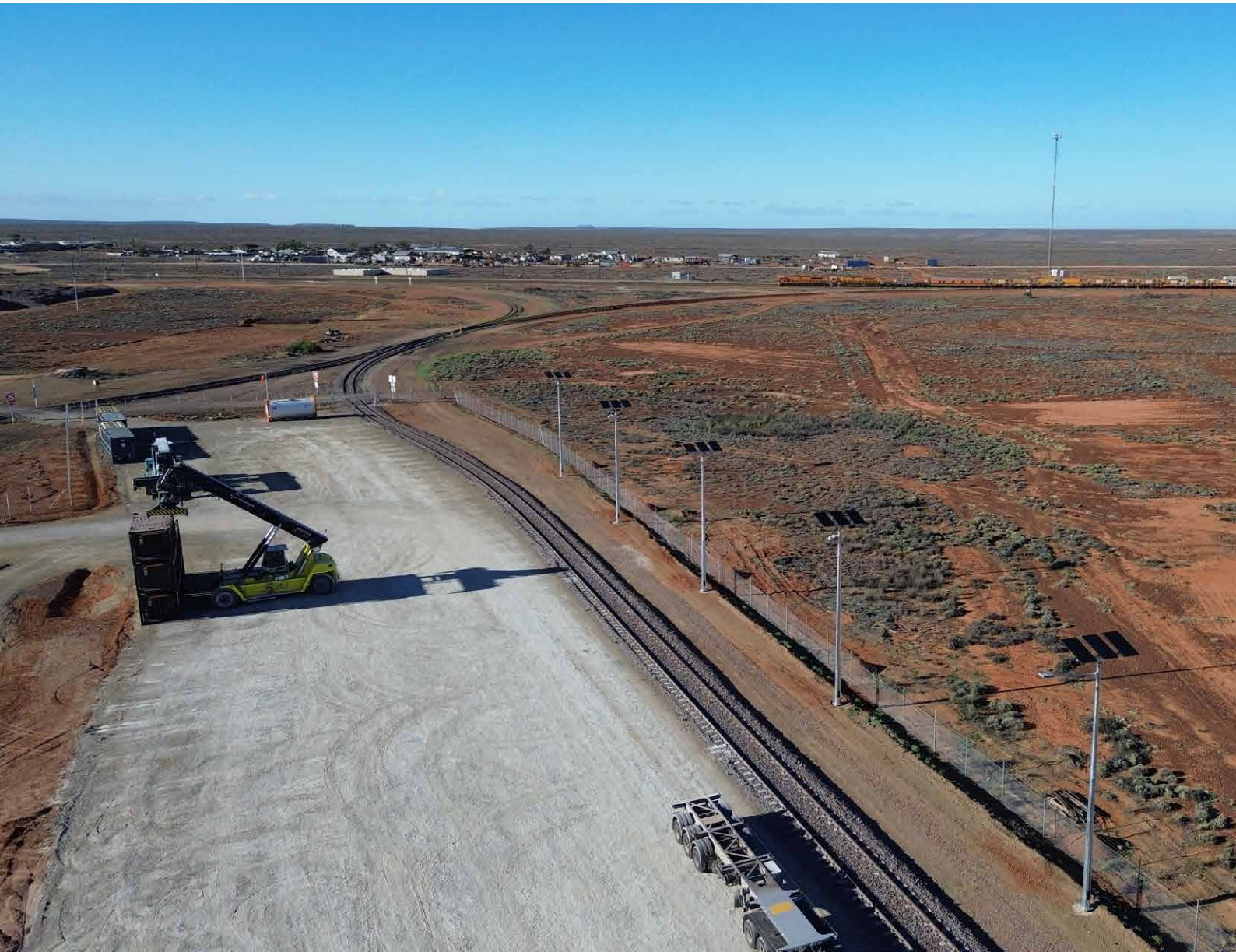
Above: Aurizon's intermodal terminal by day, showing one section of the 24 pole installation. 3 x 175W Corso Solar Engines are positioned atop each 12m pole, powering either 1 x 80W Tiger streetlight or CCTV security cameras, alternating along the length of the rail track. Below and front page: Aurizon's secure rail terminal at Pimba, South Australia, by night. 80W Tiger streetlights on 12m poles project a warm 3000K with zero upward light and minimal light spill into the surrounding terrain.
