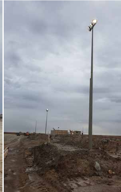
TOP: Regis Recources' Garden Well Run-of-Mine ore pad over the primary crusher, illuminated by a total of 9 high-output LED floodlights. ABOVE LEFT & CENTRE: 5 x Tiger 900W MegaFlood LED floodlights on two 15m poles positioned to illuminate the crusher, as well as the turning area & access roads. A 400W floodlight is on a shorter pole directly over the entrance to the crusher. ABOVE RIGHT: Another 15m pole carrying 3 x Primo 400W LED floods.
