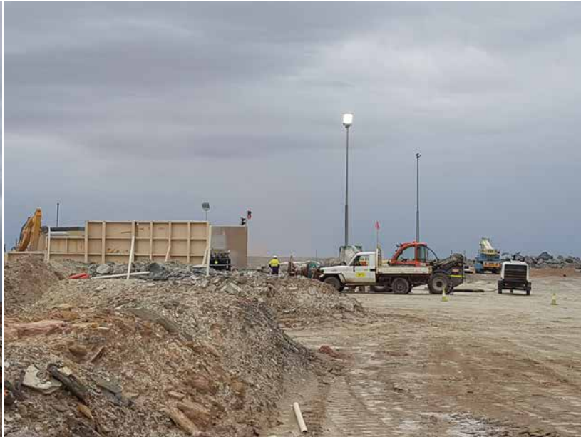
TOP: Regis Recources' Garden Well Run-of-Mine ore pad over the primary crusher, illuminated by a total of 9 high-output LED floodlights. ABOVE LEFT & CENTRE: 5 x Tiger 900W MegaFlood LED floodlights on two 15m poles positioned to illuminate the crusher, as well as the turning area & access roads. A 400W floodlight is on a shorter pole directly over the entrance to the crusher. ABOVE RIGHT: Another 15m pole carrying 3 x Primo 400W LED floods.
