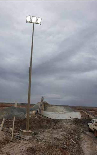
TOP: Regis Recources' Garden Well Run-of-Mine ore pad over the primary crusher, illuminated by a total of 9 high-output LED floodlights. ABOVE LEFT & CENTRE: 5 x Tiger 900W MegaFlood LED floodlights on two 15m poles positioned to illuminate the crusher, as well as the turning area & access roads. A 400W floodlight is on a shorter pole directly over the entrance to the crusher. ABOVE RIGHT: Another 15m pole carrying 3 x Primo 400W LED floods.
