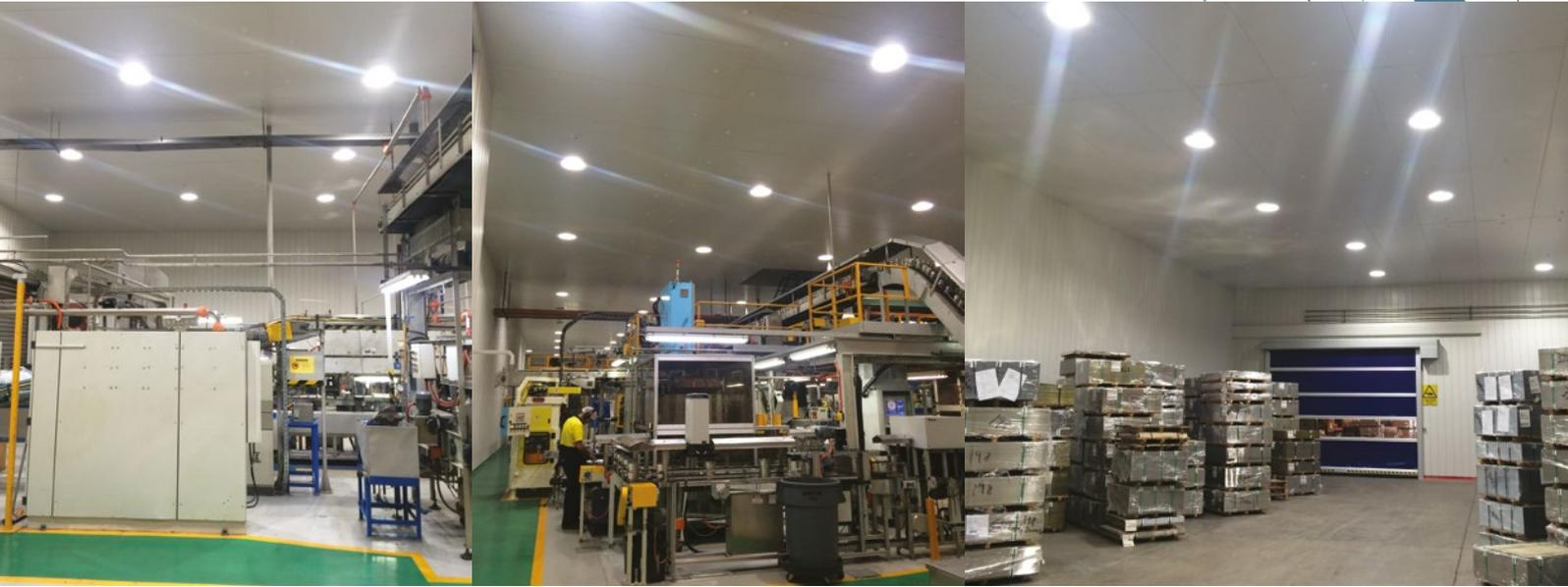
Dramatically improved lighting from the Primo 115W LED Lowbays in the ceiling panels above the manufacturing lines and adjacent raw materials bays.
