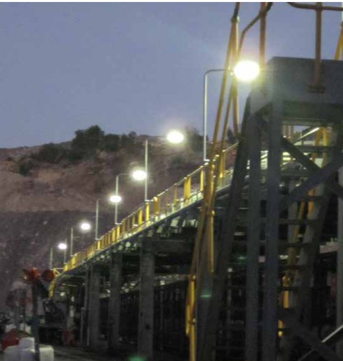
Mako 40W area lights illuminating the conveyor at Peabody Energy's Wambo Coal Mine, Warkworth, NSW.
