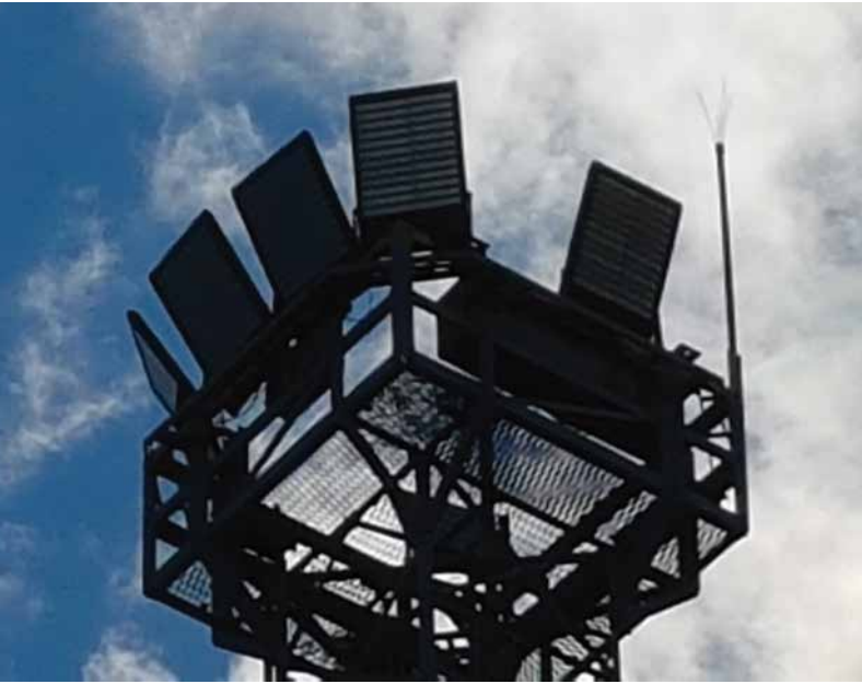
Above left and right: 6 x Tiger 900W MegaFloods on the existing 25m towers at OneSteel's Newcastle rod and wire plant.
