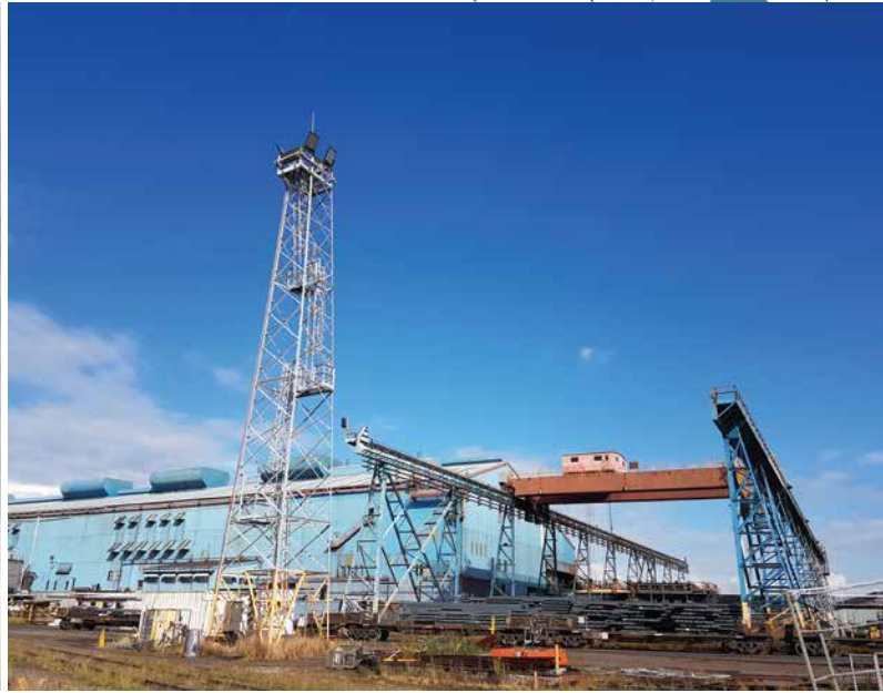
Above left and right: 6 x Tiger 900W MegaFloods on the existing 25m towers at OneSteel's Newcastle rod and wire plant.
