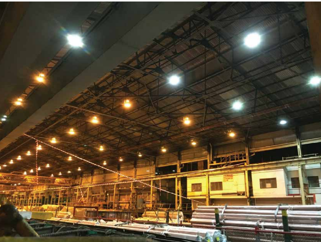
Primo 90W Lowbays being installed in the main manufacturing hall. Note the brighter whiter light from the LED lighting on the right, compared to the existing yellow sodium lights on the left..
