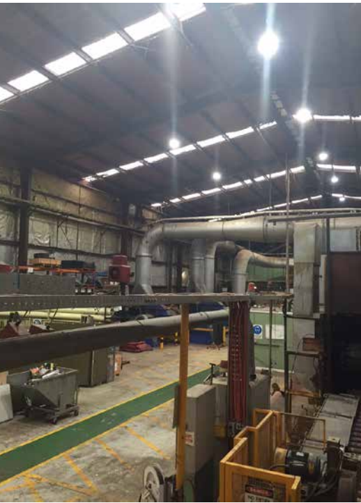
Primo 145W Dimmable LED highbays with daylight harvesting sensors at Fletcher Insulation's Pink Batt manufacturing plant at Rooty Hill, NSW.
