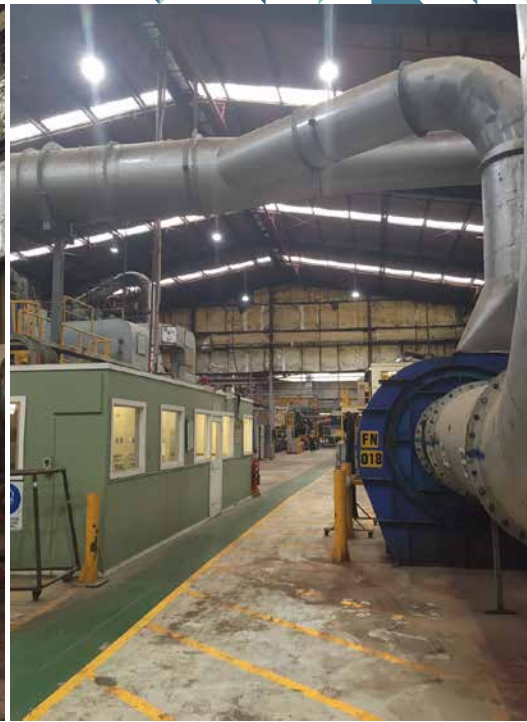
Primo 145W Dimmable LED highbays with daylight harvesting sensors at Fletcher Insulation's Pink Batt manufacturing plant at Rooty Hill, NSW.
