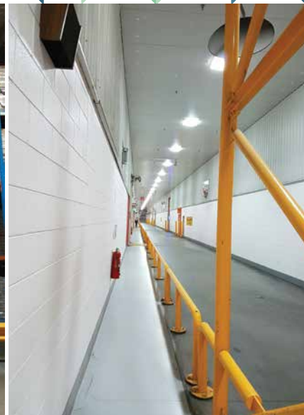
Left: Primo 90W fittings retrofitted into Wadco ceiling diffusers at 6m height in Sanitarium's packaging areas. Centre: Primo 20K LED highbays with light sensors at 10m in the Distribution Centre. Right: The "Quarter mile" passageway where older 160W LED fittings were replaced with Primo 90W low bays.
