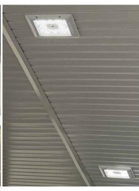
Above: 6 rows of 3 Primo 15K Canopy lights produced very impressive lux levels, with 115 degree beam spread and a bright white CCT of 5000K. Similarly, the T4M optical lensing selected for the 120W MegaFloods provided good even coverage throughout the property. Metro Petroleum sought maximum lux levels, for higher degrees of customer safety and greater efficacy of security cameras at night.
