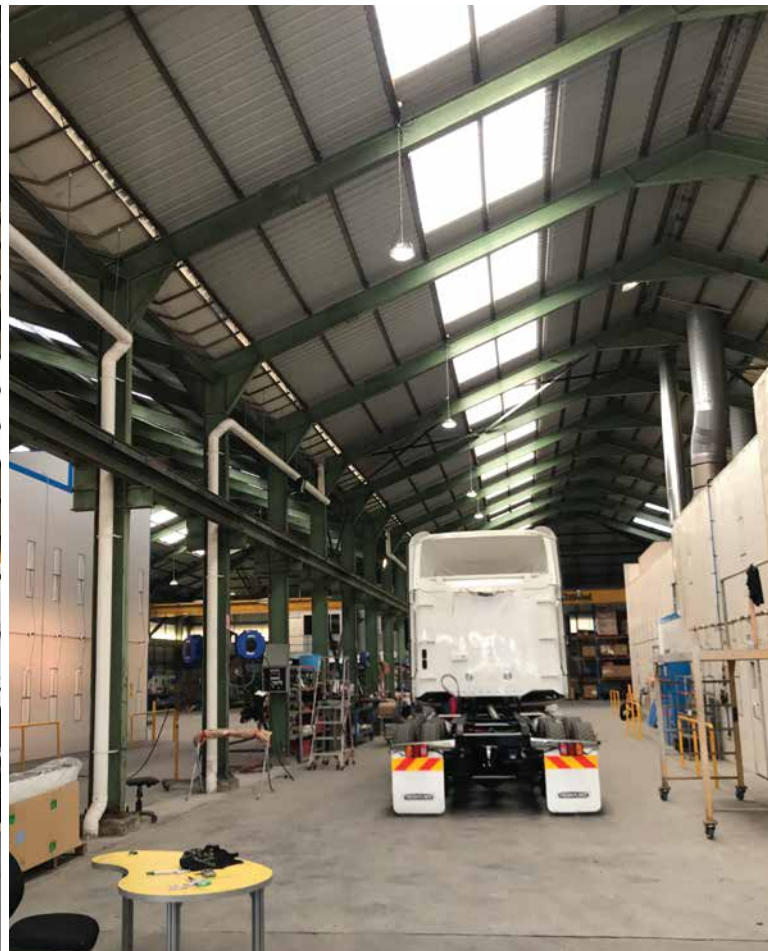
ABOVE LEFT: Primo 40K LED Highbays at 18m, illuminating the vehicle maintenance operation at Wallenius Wilhelmsen Logistics, Woolongong, NSW ABOVE RIGHT: Primo 12K Lowbays and Primo 21K Highbays in the lower ceilings at 8m. FRONT PAGE: 120W MegaFloods on walls at 6m and Primo 40K highbays in ceiling mounted at 18m, replacing 1000W MH Highbays.
