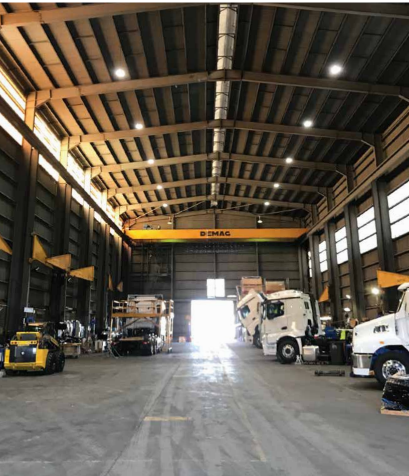
ABOVE LEFT: Primo 40K LED Highbays at 18m, illuminating the vehicle maintenance operation at Wallenius Wilhelmsen Logistics, Woolongong, NSW ABOVE RIGHT: Primo 12K Lowbays and Primo 21K Highbays in the lower ceilings at 8m. FRONT PAGE: 120W MegaFloods on walls at 6m and Primo 40K highbays in ceiling mounted at 18m, replacing 1000W MH Highbays.
