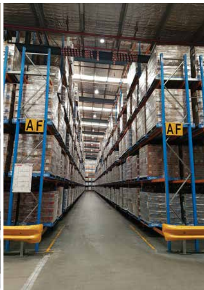
Left: Primo 90W fittings retrofitted into Wadco ceiling diffusers at 6m height in Sanitarium's packaging areas. Centre: Primo 20K LED highbays with light sensors at 10m in the Distribution Centre. Right: The "Quarter mile" passageway where older 160W LED fittings were replaced with Primo 90W low bays.
