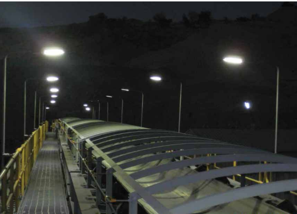
Mako 40W area lights over the conveyor at Peabody Energy's Wambo Coal Mine, Warkworth, NSW.
