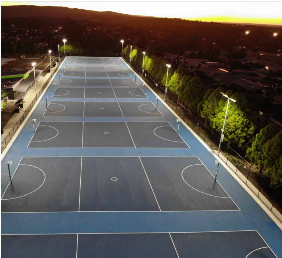
Excellent uniformity of light distribution over the 10 courts at the Newborough courts, with minimal light spill into surrounding areas. The Show-court is the second court from top, above left, utilising 1440W Striker fittings, which can be dimmed when 350 lux ave is not required.
