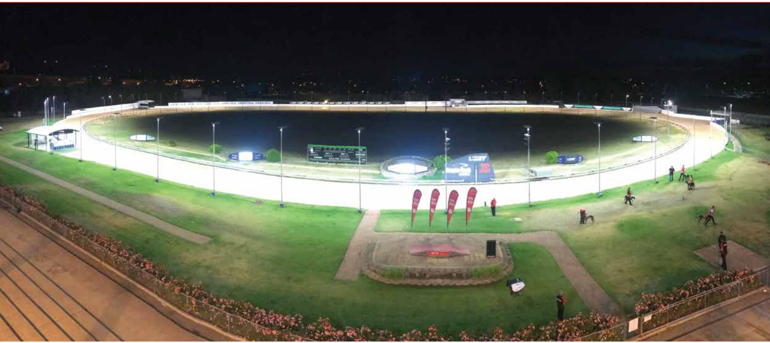
Above and right: Brilliant, uniform light from Tiger 600W MegaFloods spigot-mounted on existing 8m poles at Angle Park, SA. [Note old 1500W MH floodlights on far side of track.]
