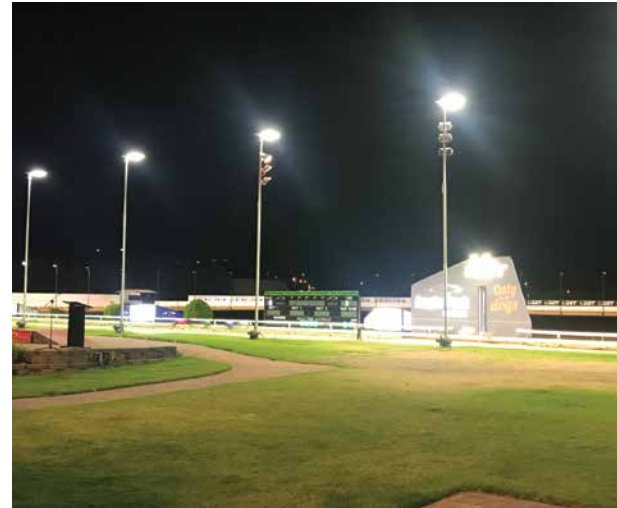
Above and right: Brilliant, uniform light from Tiger 600W MegaFloods spigot-mounted on existing 8m poles at Angle Park, SA. [Note old 1500W MH floodlights on far side of track.]
