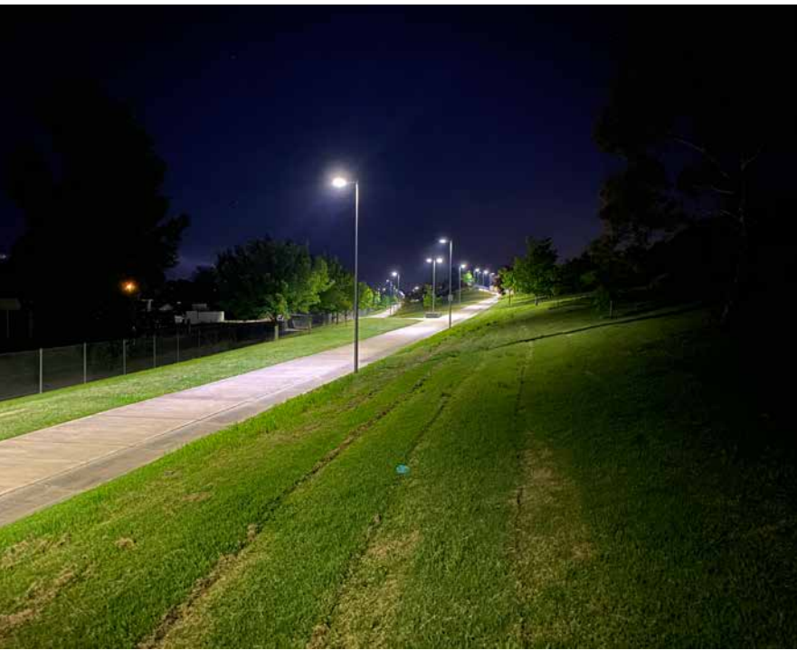
Excellent uniformity with minimal obtrusive light spill along the 10.4km track.
